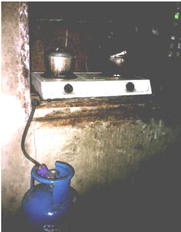
Photo 5. A typical LPG cooking stove with bottled gas, a system used in more than 4 million households in the Philippines.
