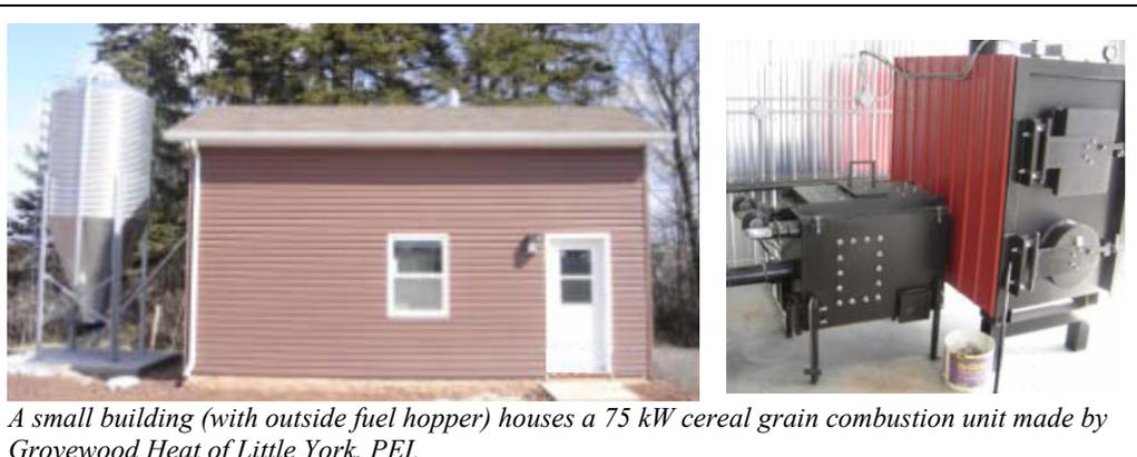
*A small building (with outside fuel hopper) houses a 75 kW cereal grain combustion unit made by Grovewood Heat of Little York, PEI.*
